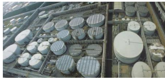
Wastewater treatment plant (after improvement)
