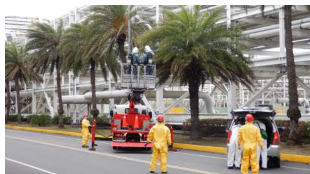
Expand drills for public pipes
